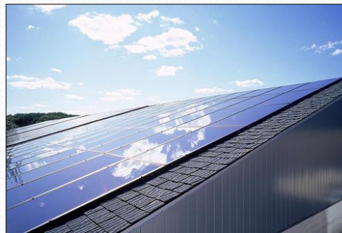
Solar roof panels
